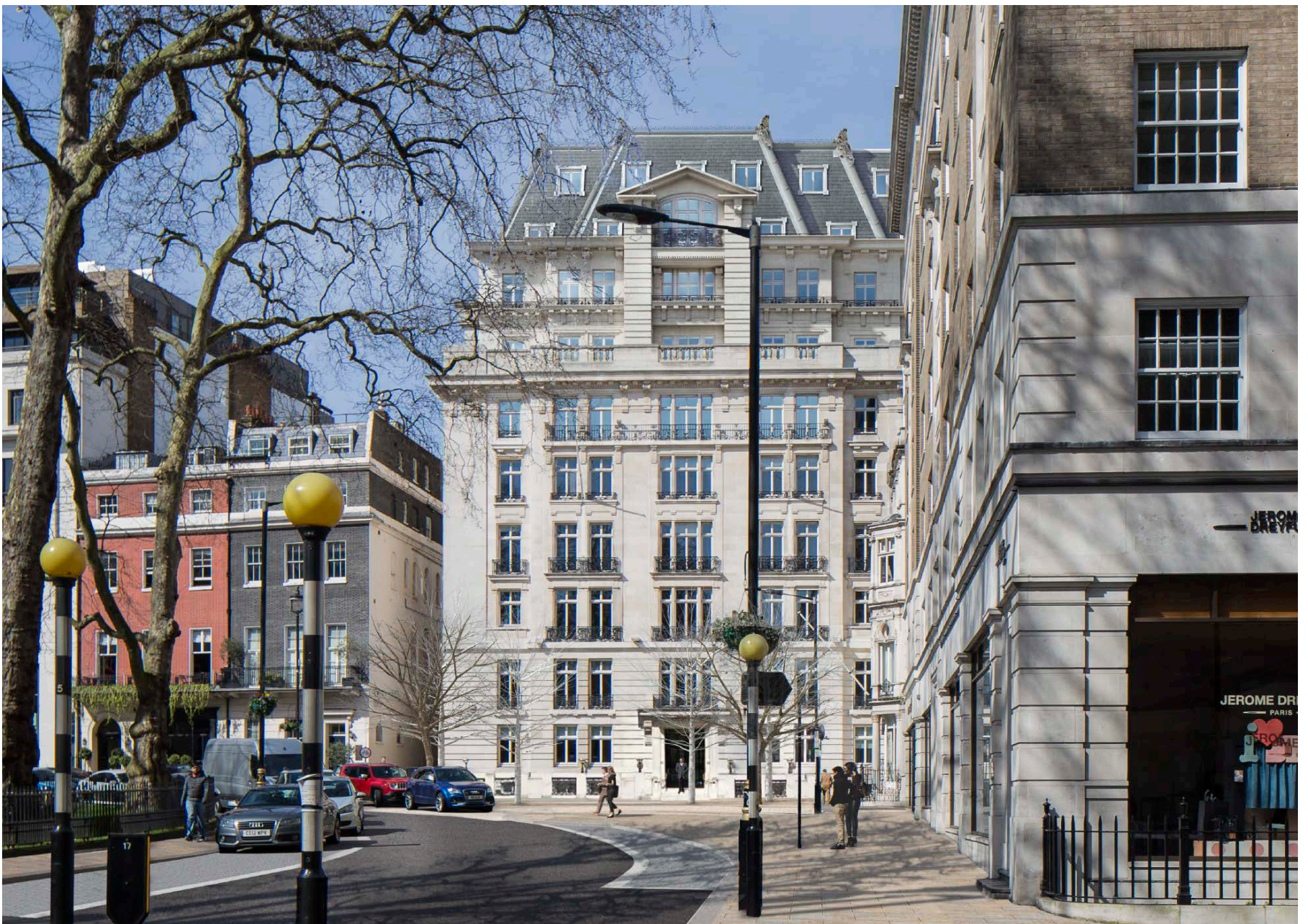
South facing and occupying the north east corner of the Square, N°25 directly overlooks the gardens. Current public realm enhancements to Berkeley Square allow for a number of improved streetscape works.
